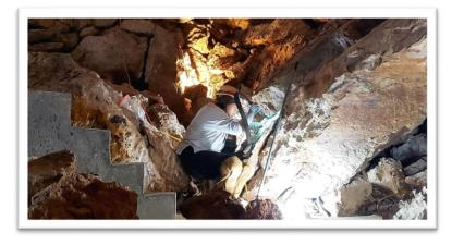
Walkways constructed of decking material are being replaced with concrete that provides better footing and steel handrails. A new route has eliminated seven steps and allows guests to walk amongst the rocks rather than above them. Extreme care was taken to ensure that no living cave formations were damaged in the process of building the pathway. To protect the air inside the cave from dust, a double tent houses portable concrete mixers and bagged concrete that's mixed by hand in small batches.
